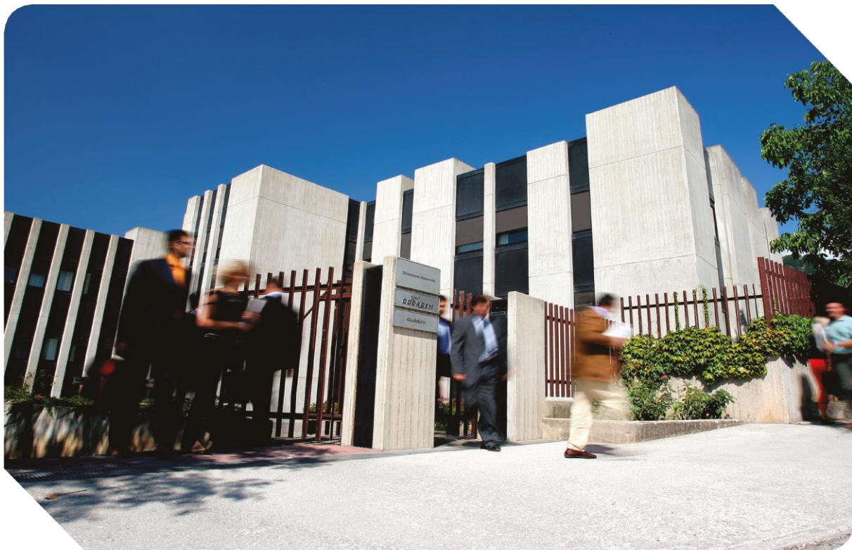
Figure 1 – Headquarters of Colacem S.p.A. - Gubbio (PG)
